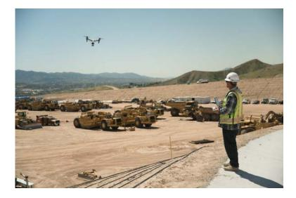
Instead of creating a topo of the site using a GPS rover, which would have required the grade setter to walk on steep slopes and shoot points by hand, **the grade setter flew a drone** to collect hundreds of photos that would be uploaded to the TraceAir platform to create a digital copy of the site. A single drone flyover took a few hours to complete, **allowing the team to see a near real-time 3D map in under 24 hours**, twice a week.
